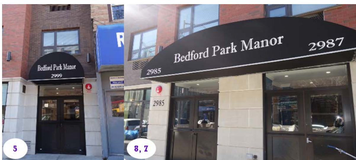
The Webster Avenue Vision Plan and Rezoning spurred housing development on the Webster Avenue boundary of Bedford Park.
