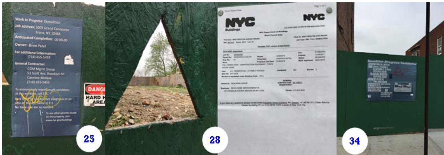
Demolition of 1-to-4 Family Homes
